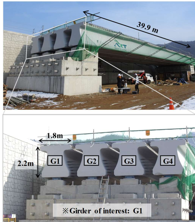
(a) Bridge under construction (December 19, 2017)
