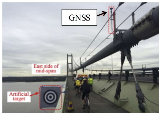
(b) Humber Bridge in Hessle and Barton, United Kingdom [109]
