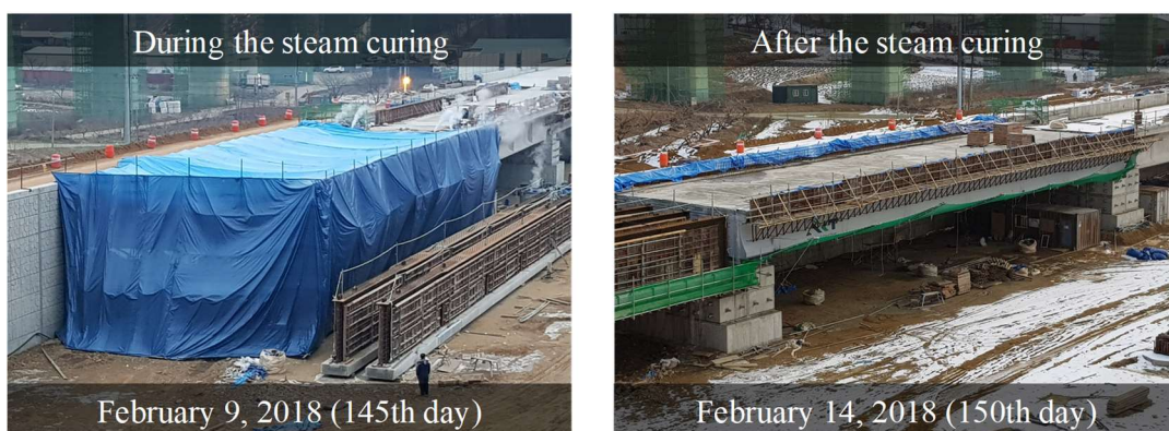
Figure 46. Construction site during and after the steam curing.
