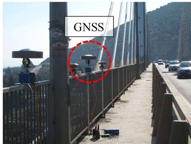
(a) Evripos bridge in Halkida, Greece [108]
